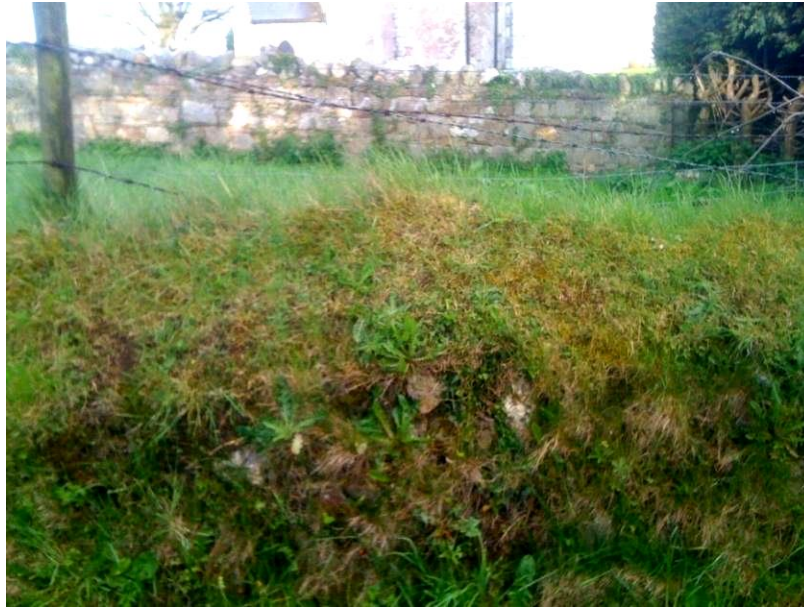
Fig. 16 Close up of the earth bank next to the Church of Ireland
