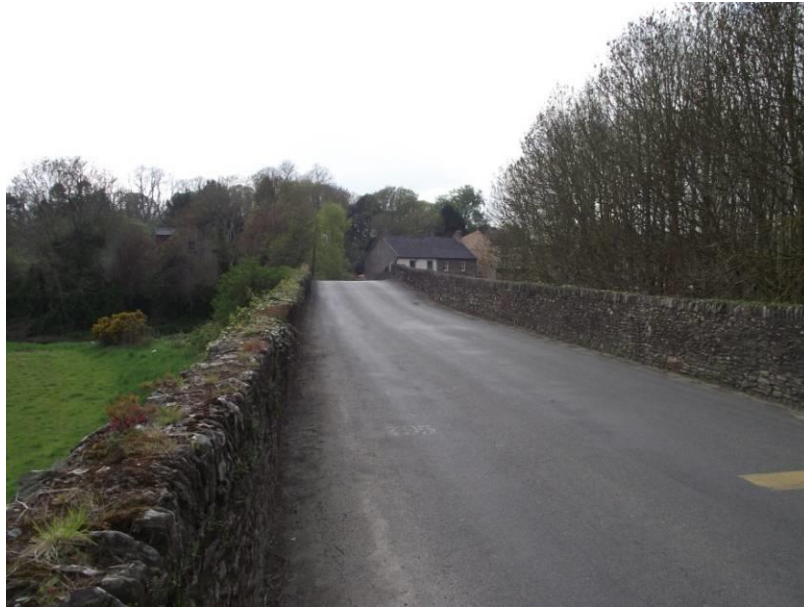
Fig. 18 Limestone Bridge over the River Derry
