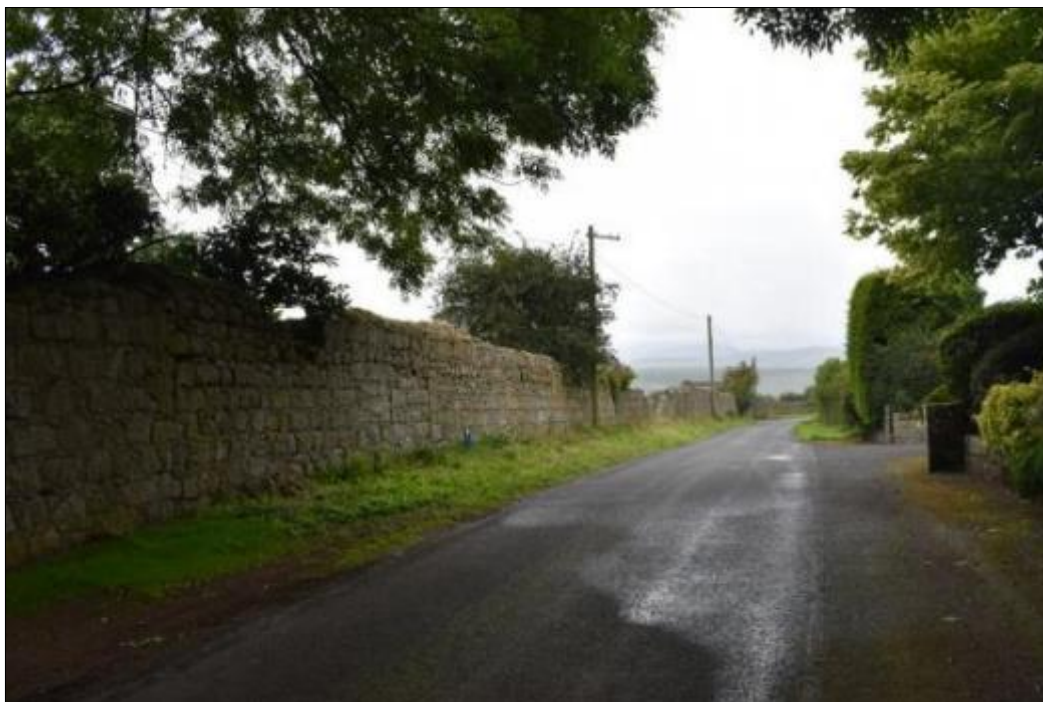
Figure 100 Granite estate wall, Kilbride townland
