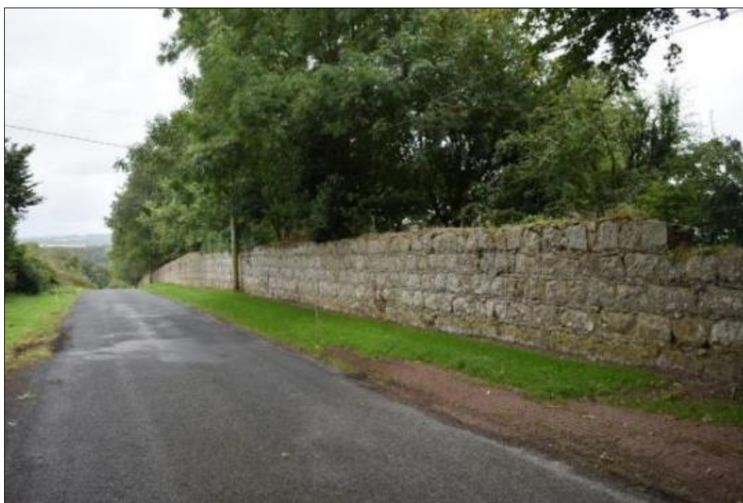
Figure 101 Granite estate wall, Kilbride townland
