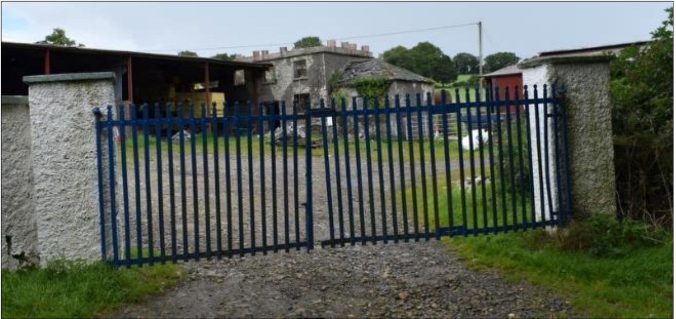
Figure 121 Double iron gate in Ballinvally townland
