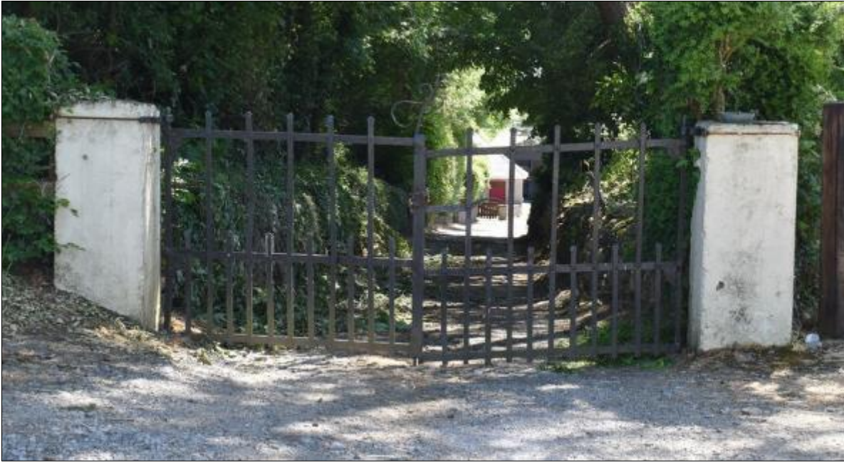
Figure 120 Double iron gate in Barragh townland
