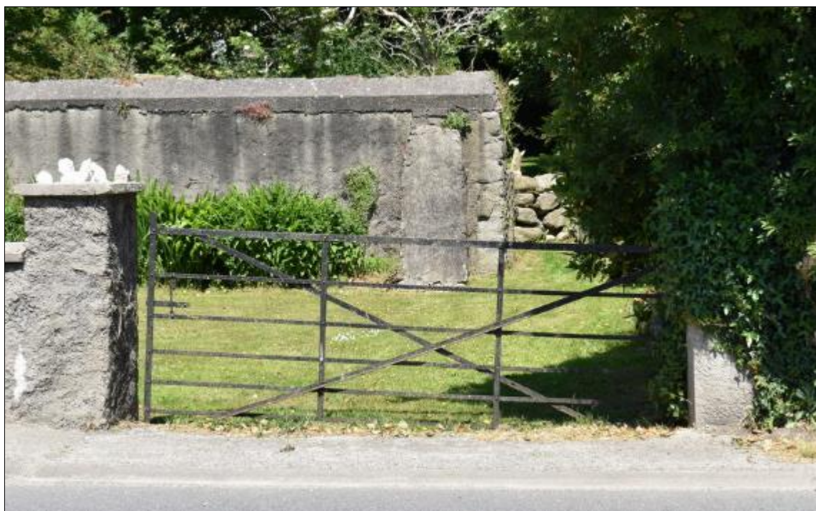
Figure 119 Iron gate Kildavin village
