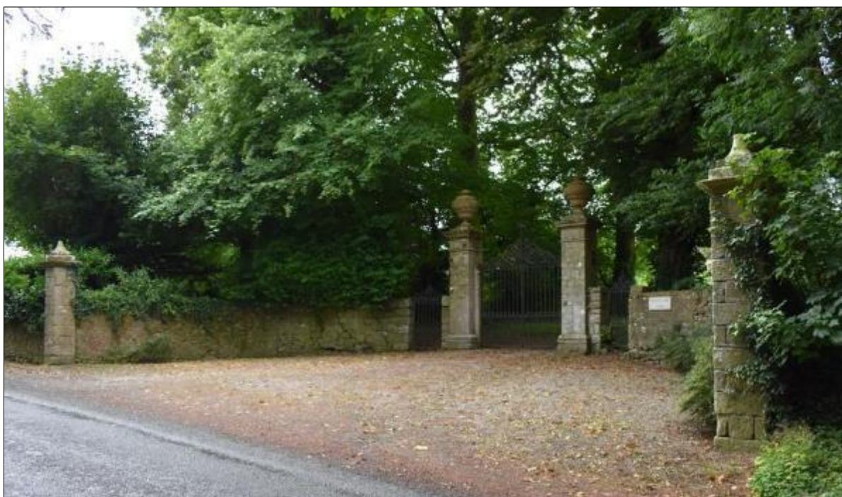
Figure 95 Entrance to Sherwood Park House
