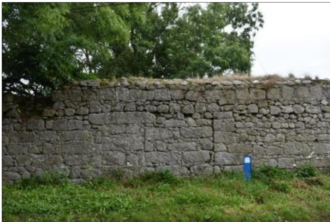
Figure 102 Granite estate wall, Kilbride townland
