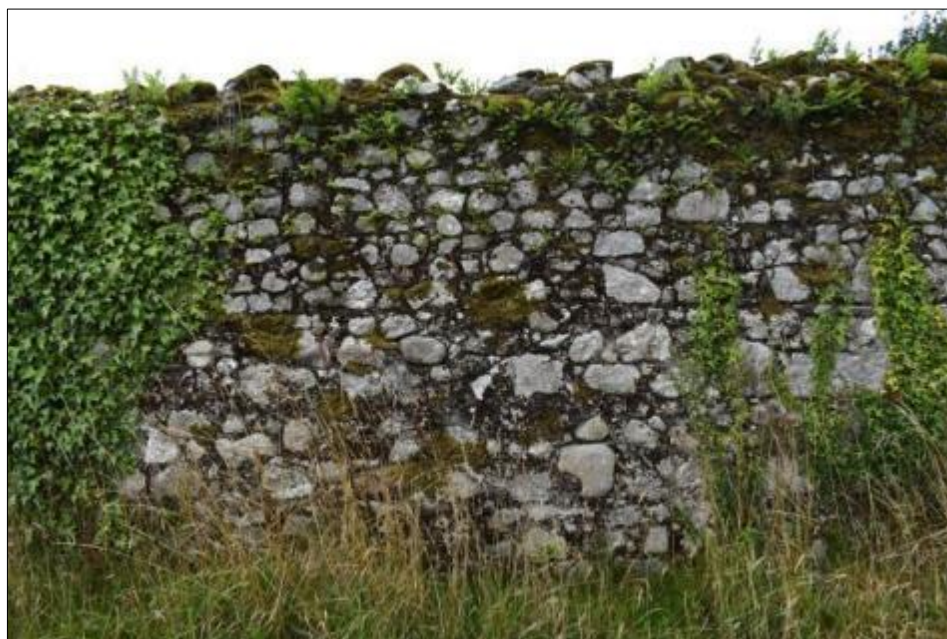
Figure 105 Granite estate wall, Sherwood Park
