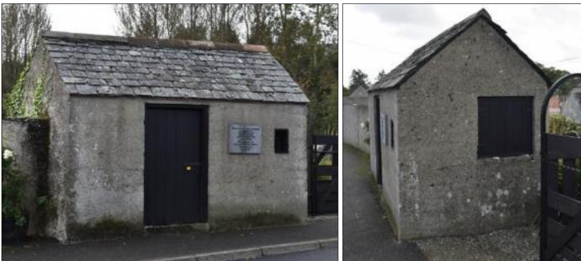
Figure 13 Old weighbridge building
