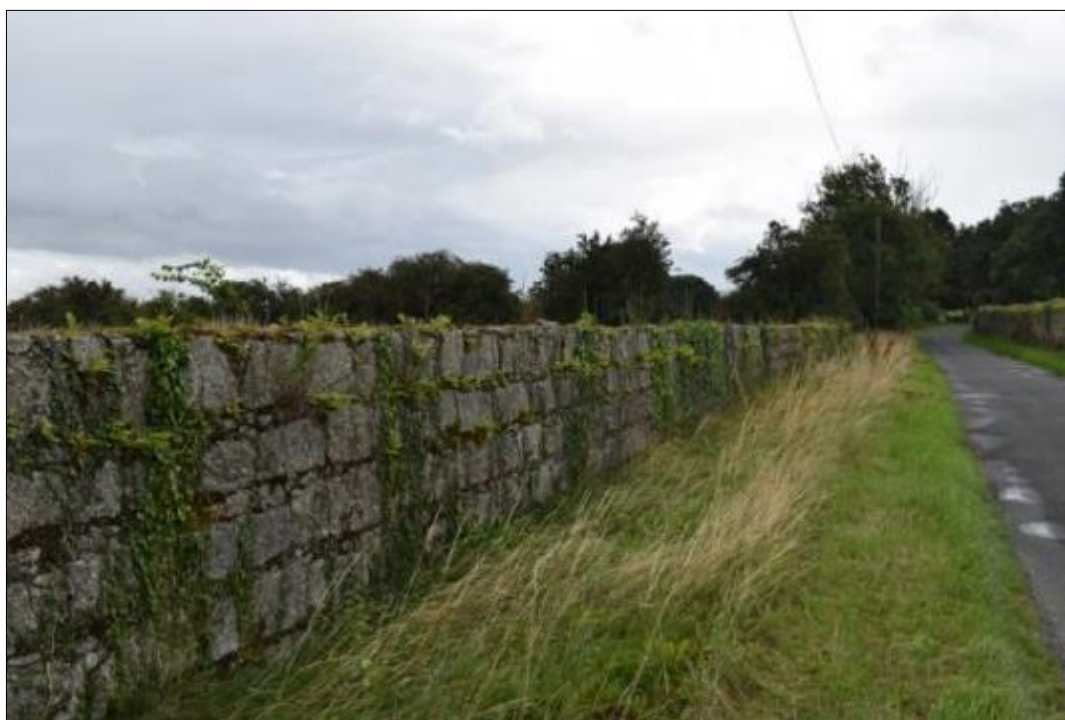
Figure 103 Granite estate wall, Kilbride townland
