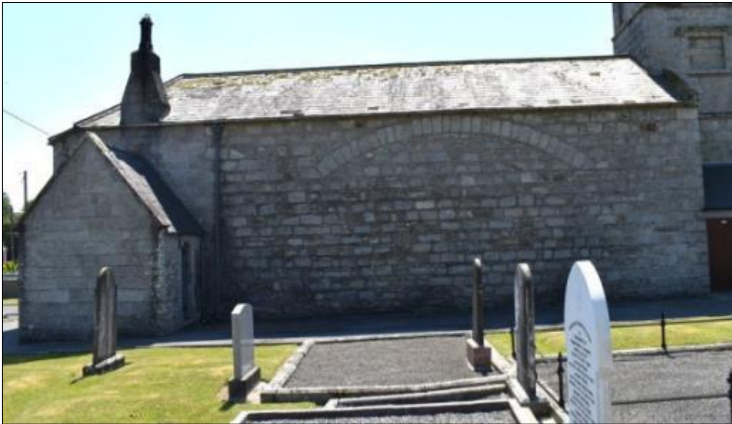
Figure 88 Relieving arch in the northern wall of St. Paul's church
