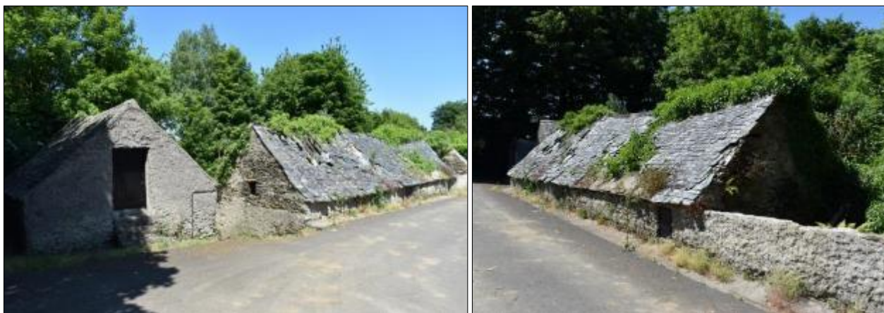
Figure 110 Vernacular farm building at Ballypierce
