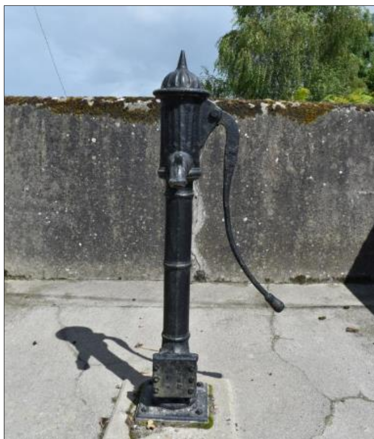
Figure 147 Water pump, Crowsgrove
