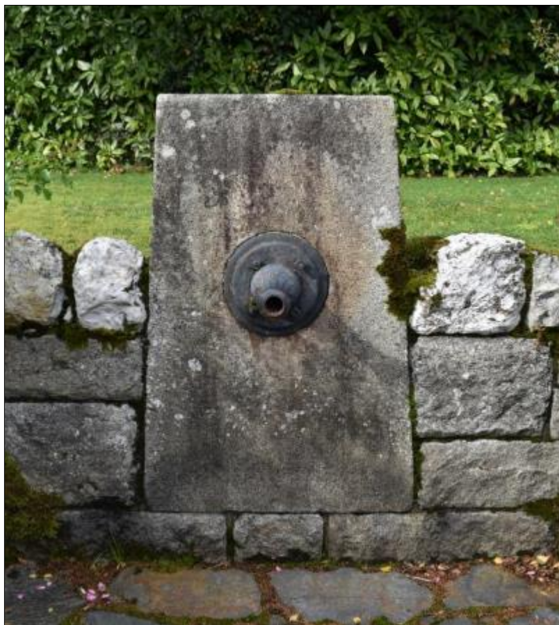
Figure 152 19th century water spout at Carrickduff
