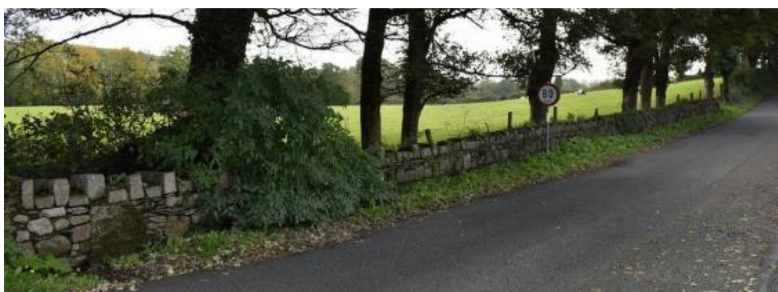
Figure 21 Stone wall along the southern side of the village
