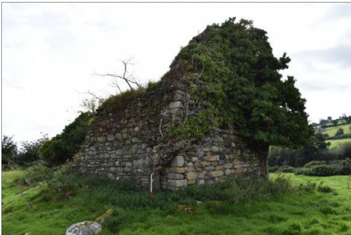
Figure 42 Barragh church, looking southeast
