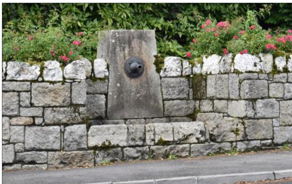
Figure 153 19th century water spout at Carrickduff
